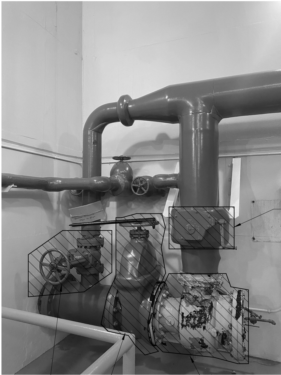
REPLACE EXISTING 6" GATE VALVE WITH 6" GATE VALVE w/ PNEUMATIC ACTUATOR REPLACE EXISTING 14" GATE VALVE IN KIND REPLACE EXISTING 12" MANUAL BUTTERFLY VALVE IN KIND REPLACE EXISTING 10" SURGE RELIEF VALVE IN KIND
